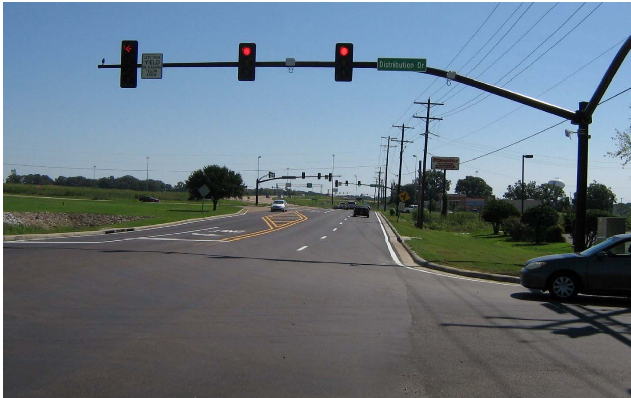
Looking east on Gluckstadt Road at Distribution Drive
