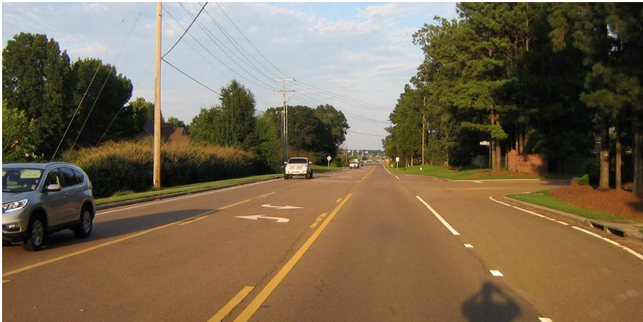
Below – Looking east on Gluckstadt Road at Planters Row
